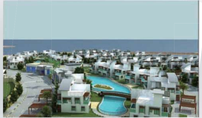
Aerial View (Waterfront Villas)
